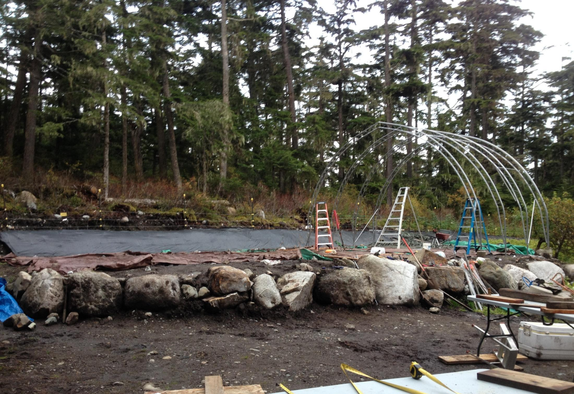
Setting arches in place: cross braced end arches
