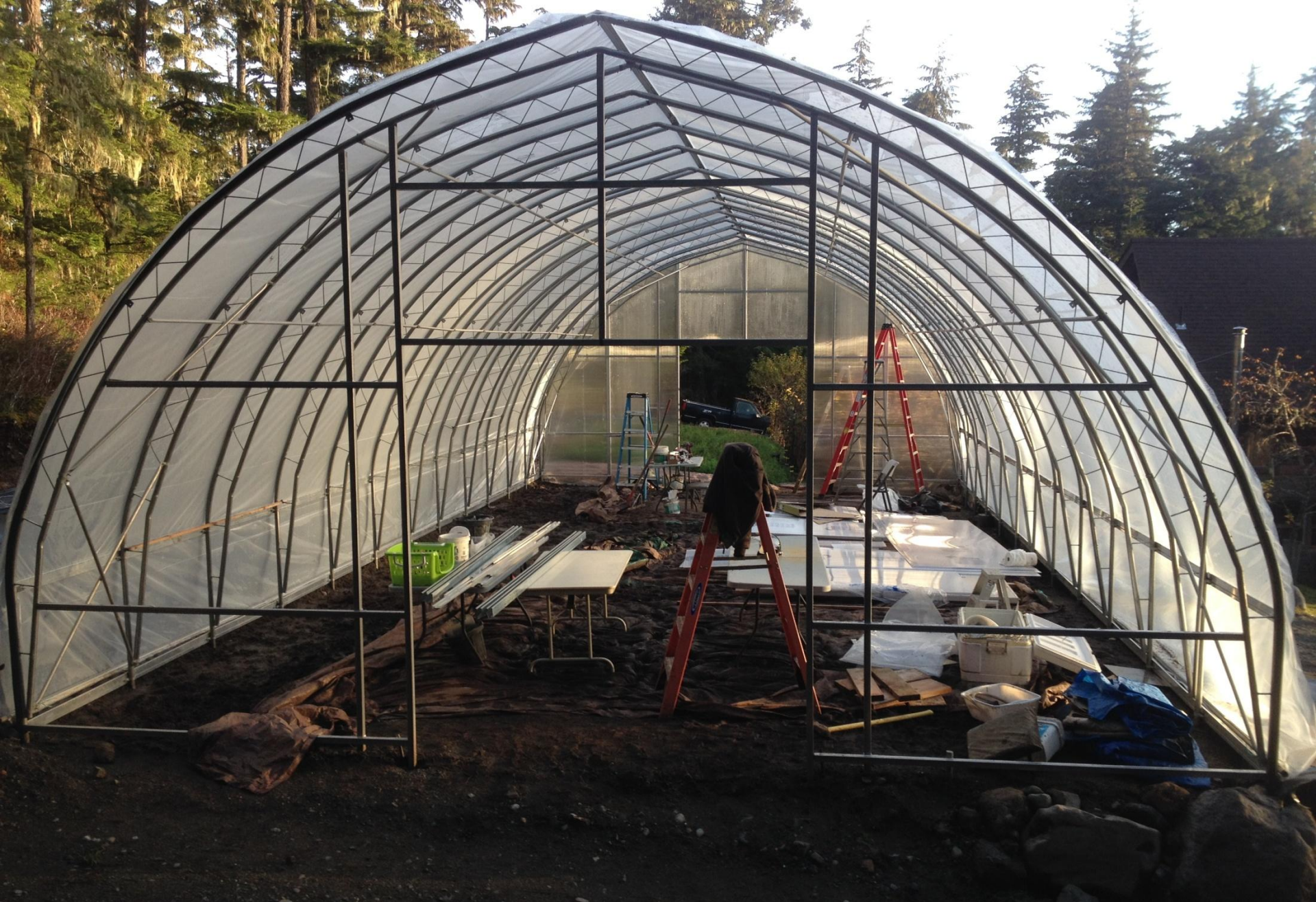
Framing end walls
